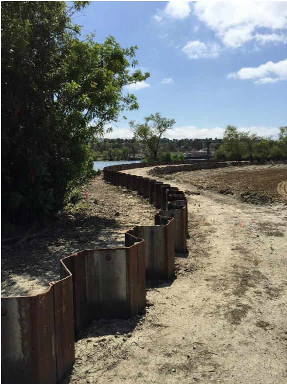
HOT ROLLED with Larssen Interlock
