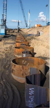
A Combined Wall (also referred to as a "Combi-wall") is a structural design for a bulkhead wall using a combination of pipe, beams, and/or sheetpiling that are connected with interlocks in order to provide a very high strength alternative to typical sheetpiling designs.
